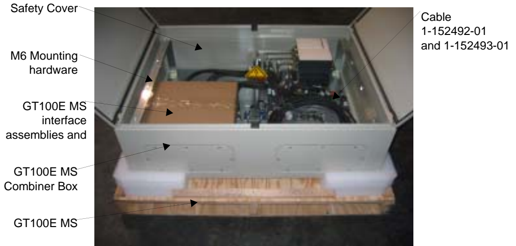
Figure 2-1 GT100E MS Components
